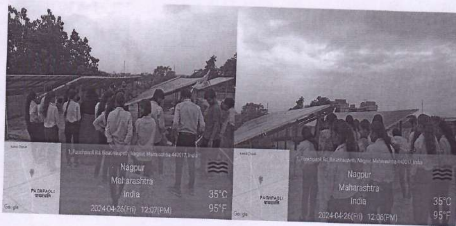
Mr. Vikas Mishra explained about Installation of Solar Panel
