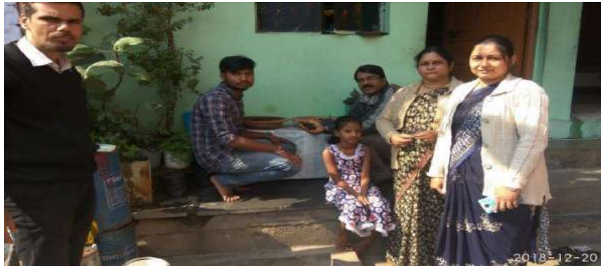
Portable Pit installed at students house
